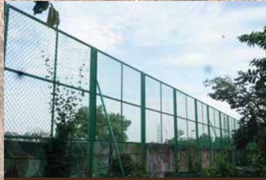
The fence on the western boundary
